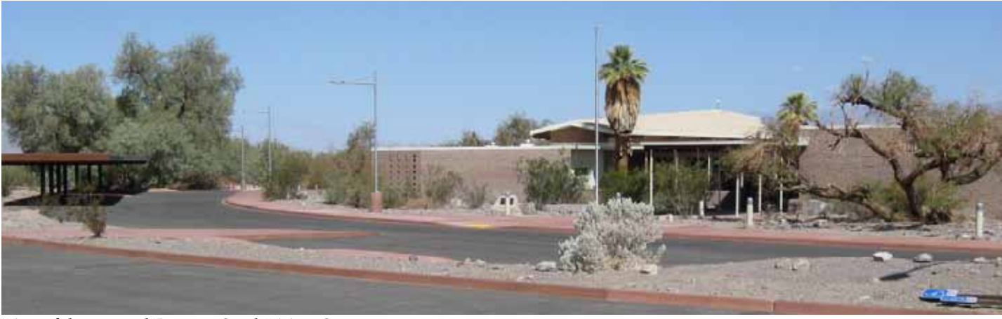
View of the restored Furnace Creek Visitor Center
