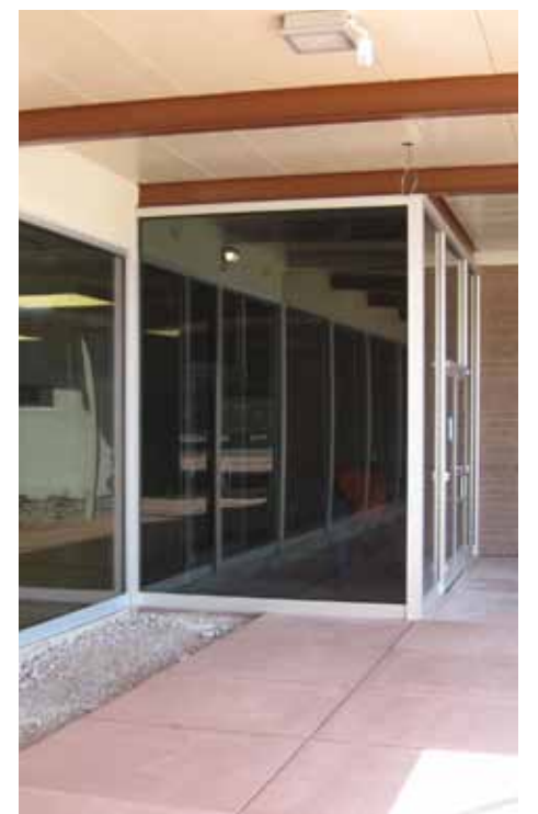
New energy saving air-lock entry to the Furnace Creek Visitor Center
